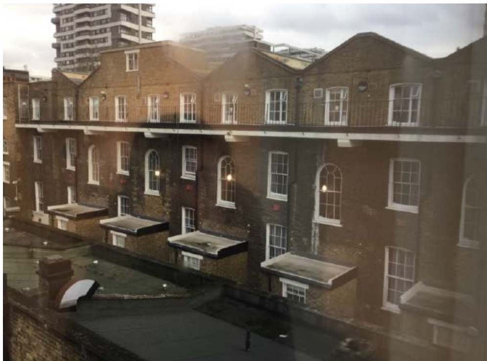
View of roofs of application site with Wilson House student halls of residents behind.
